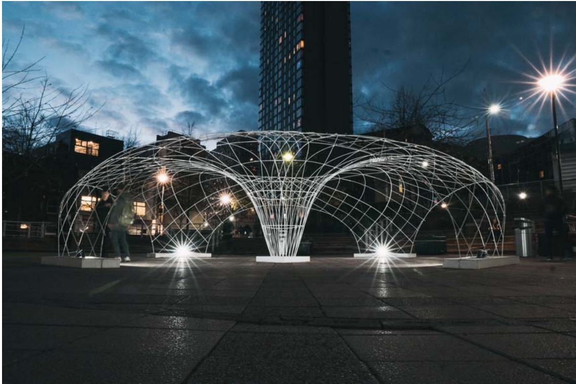
Figure 1: Final structure erected in November 2016 at Hallam Square, Sheffield, UK (© Matt Bell for SHU)
