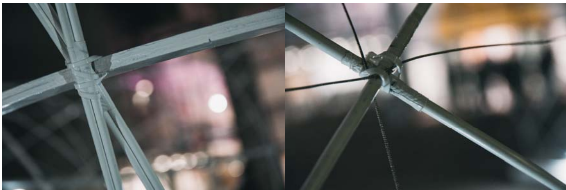
Figure 9 Rods to rings, and rods to cable connection details using gaffer tape and cable ties (© Matt Bell for SHU).
